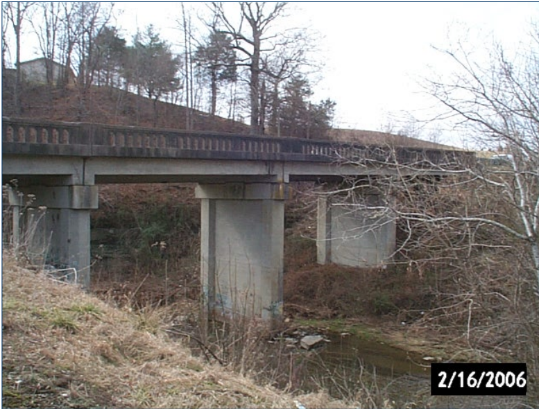
Photo 34 Dutch Creek Bridge and KY 90.
