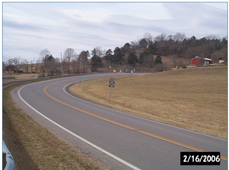
Photo 41 Westbound KY 90 approach to KY 691 intersection. Sharp curve, uphill, limited visibility.
