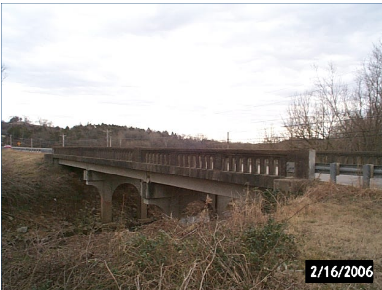
Photo 36 Allen Creek Bridge and KY 90.
