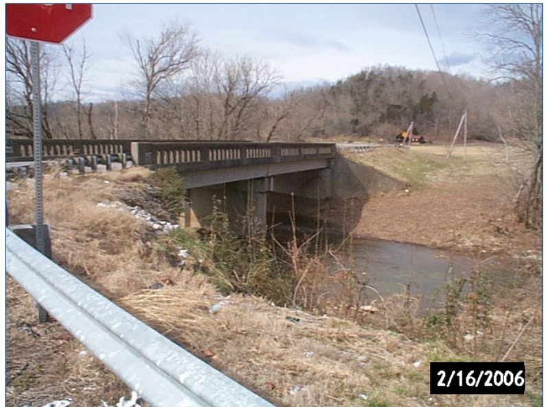
Photo 29 Wisdom Creek Bridge and KY 90.
