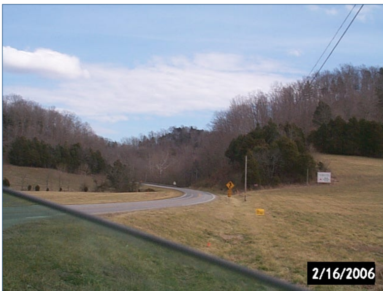
Photo 42 Eastbound KY 90 approach to Burkesville Hill Road/Saw Mill Cut. Sharp curve, uphill, limited visibility.
