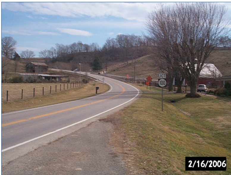
Photo 30 Eastbound KY 90 approaching KY 100 intersection. Sharp curve, limited visibility, KY 100 intersects at an oblique angle.
