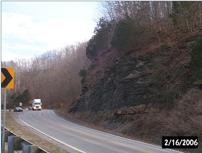
Photo 46 Westbound KY 90 on Burkesville Hill. Deep rock cuts.
