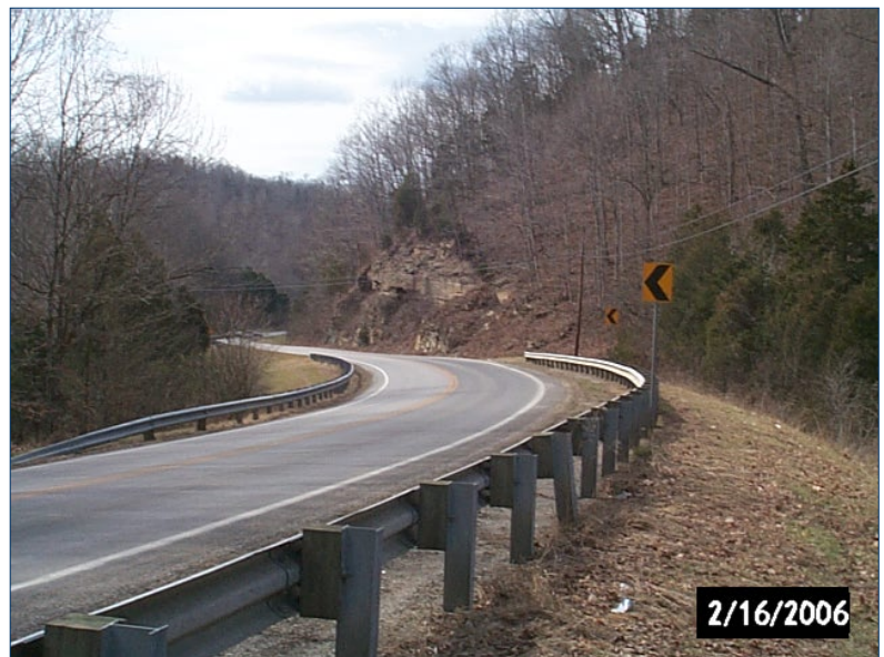
Photo 47 Westbound KY 90 on Burkesville Hill. Sharp curve. deep rock cuts.
